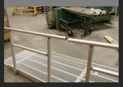
12. Mount the bottom and upper part of the handrail and tighten the screws.
