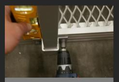
14. Plumb the rail. Tighten the screws for the railholder, always tighten the left screw first.
