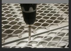
7. Use the pervading screw with associated nut and washer on the bottom between the ramp sections.
